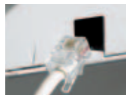
Telephone plug at the base of the door phone.
