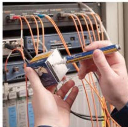
removed. If necessary, repeat your cleaning steps to remove any lingering soils not removed by the first cycle.
